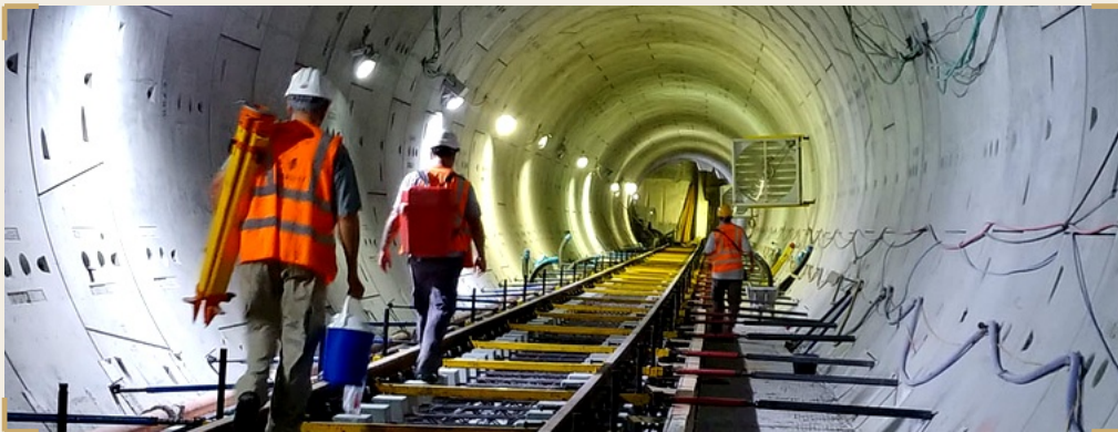
Israel light rail tunnel, AZ Marketing Group project
